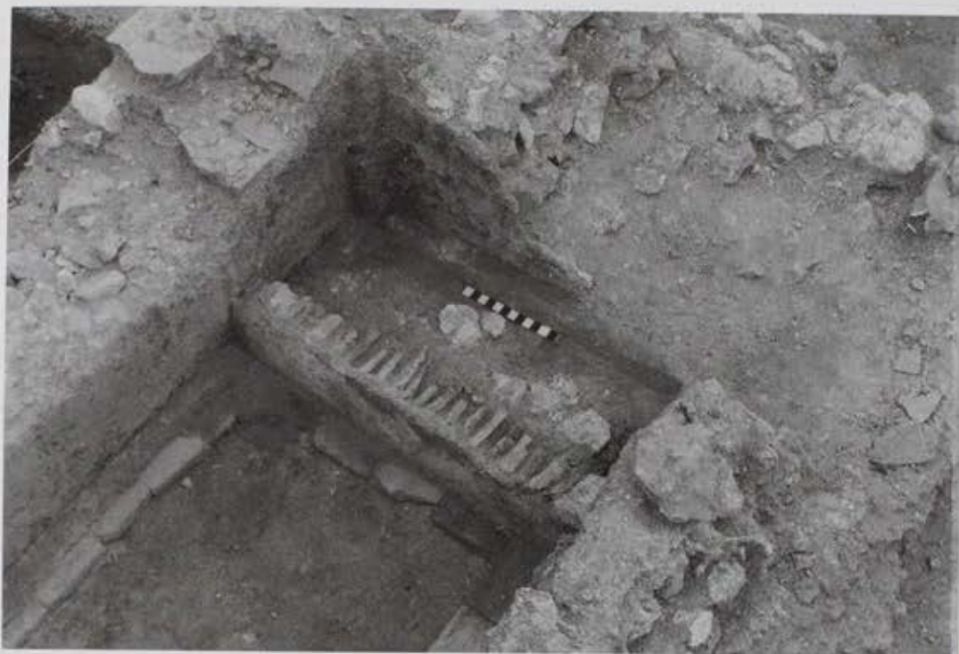
Fig 34 View of the tiles used in the construction of the steps into the bath in Room 18 (photographed 1972)
