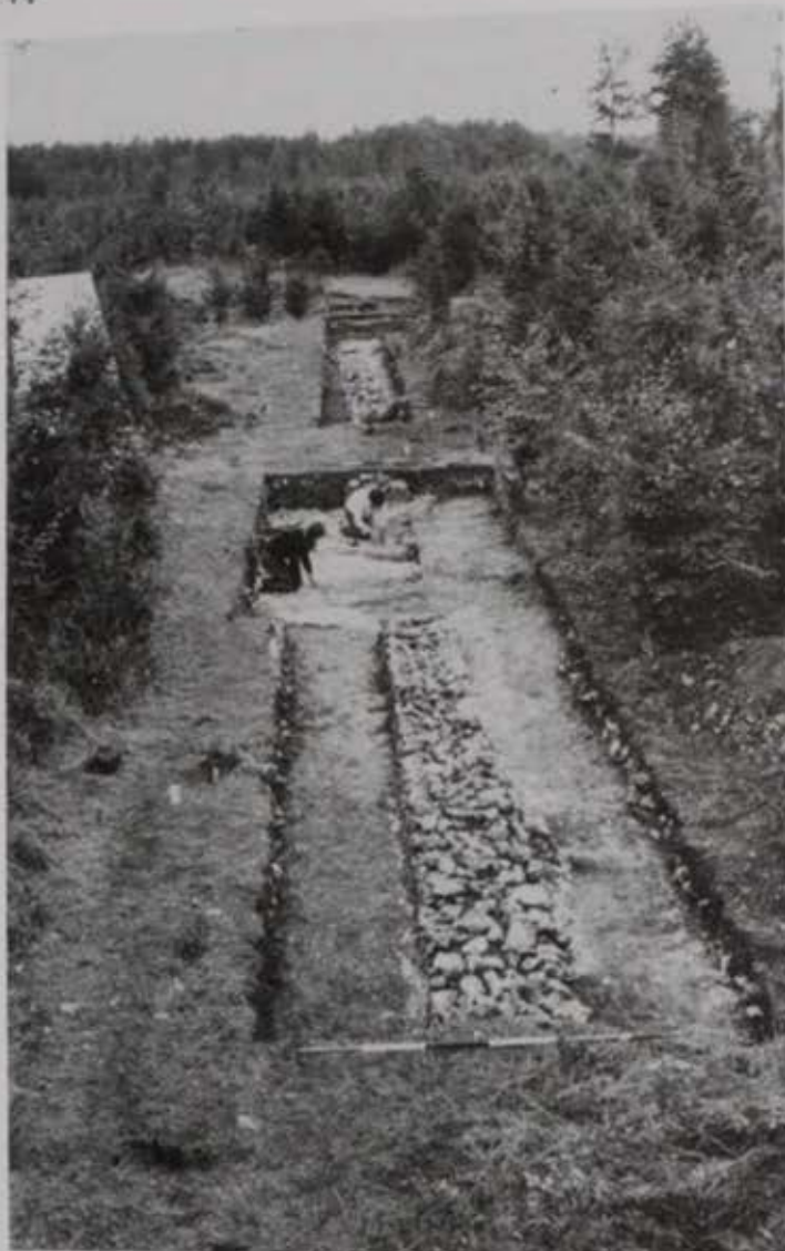
Fig 74 Eastern wall under excavation (photographed 1968)
